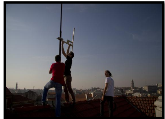
Photo 13: Members of Radio Zero hoist antenna for Future Places broadcast
